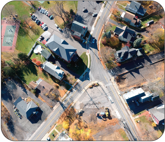
above: Community Day 2023 below: Voorheesville intersection of The American Legion Post, Nichols Park and Voorheesville Village Hall, as well as the future home of the Blackbirds Restaurants, as seen from above.
